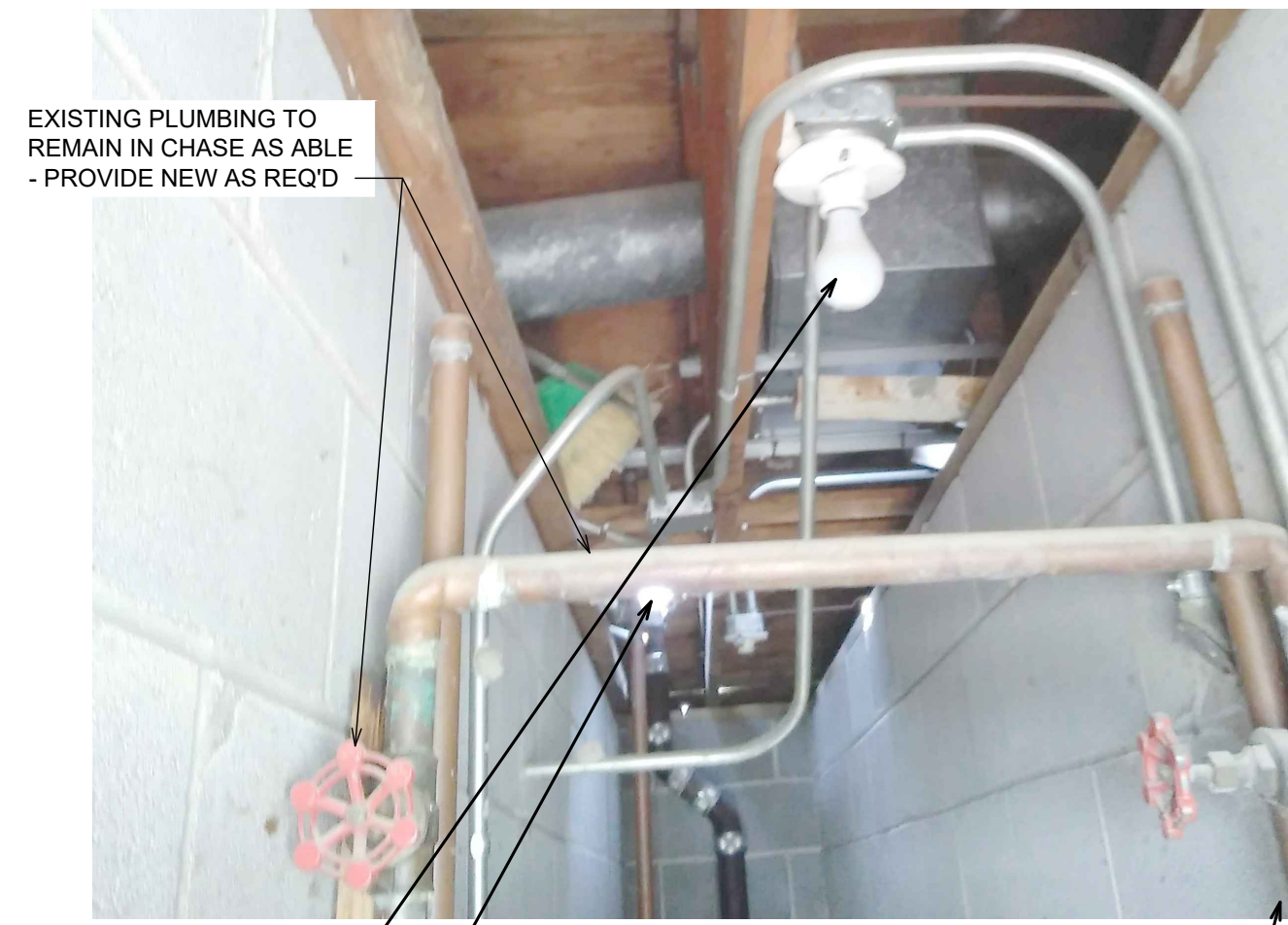
RELAMP EXISTING SOCKETS WITH NEW CFL LAMPS - REPLACE NON-FUNCTIONING DEVICES AS REQ'D (TYP.)
