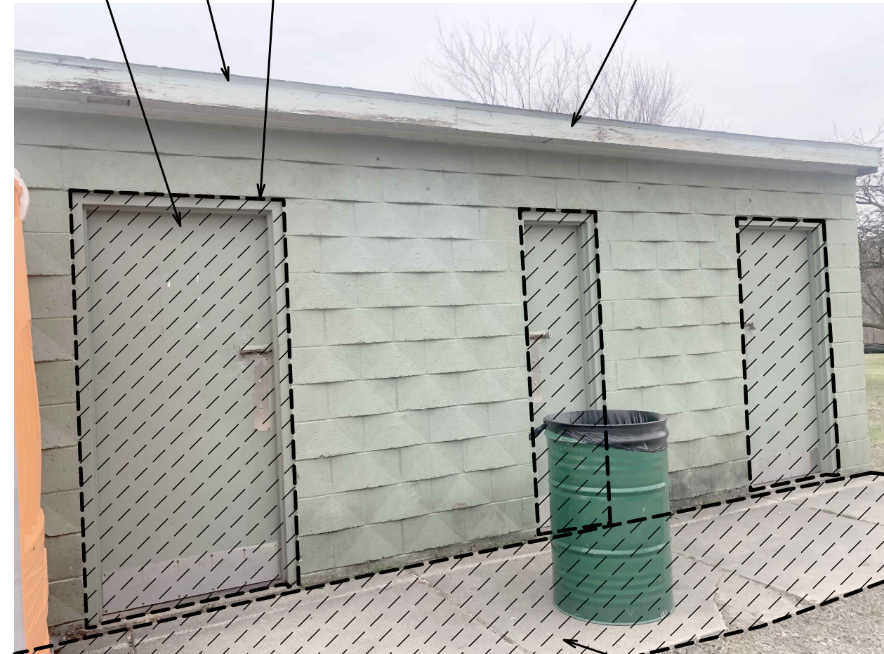
REMOVE AND REPLACE CONCRETE SIDEWALK. MATCH FOOTPRINT OF EXISTING. REFER TO DETAIL ON SHEET G-2. MAINTAIN ADA SLOPES WHERE CONNECTING TO EXISTING PAVING.
